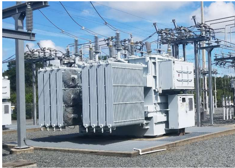
Fig. 2.3. A distribution transformer in a substation. Photo by B. Ross.
