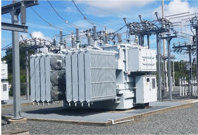
Fig. 2.3. A distribution transformer in a substation. Photo by B. Ross.
