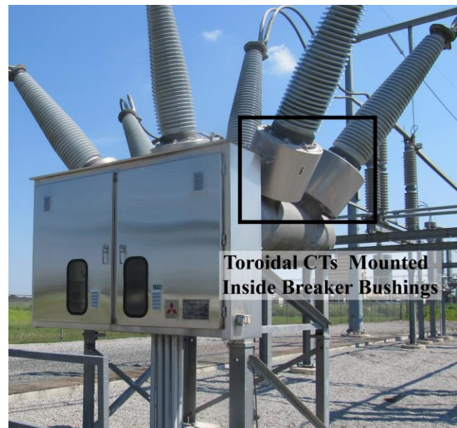
Fig. 3.6. 230kV gas-insulated breaker with bushing mounted CTs. Photo by B. Ross.
