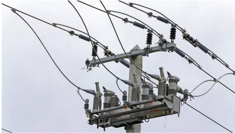
Figure 27: Recloser in a Distribution System
