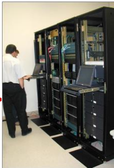
SCADA Master Station
